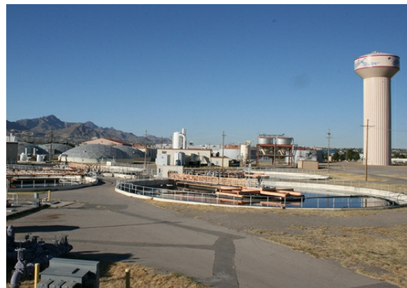
Haskell R. Street Wastewater Treatment Plant built in 1923.
