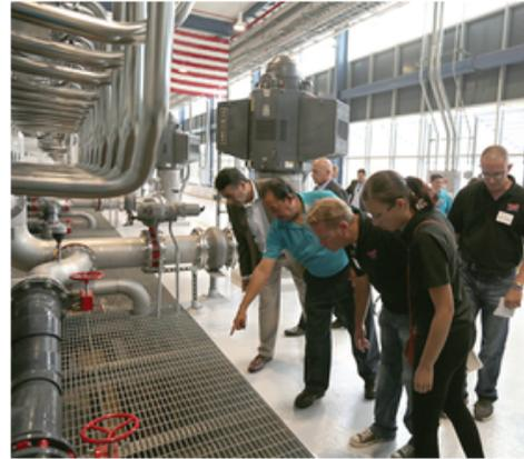
Water plant Senior Technician Jose Ronquillo (*second from left*) shows feed water piping that feeds the reverse osmosis booster pumps at the KBH Desalination Plant.
